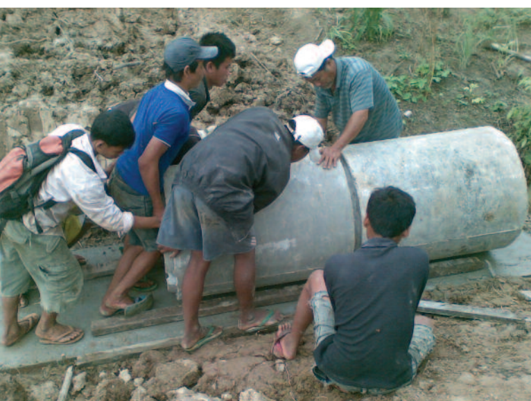
Drain construction, Pha Tad Ke Botanic Garden. (Image: Rik Gadella)
