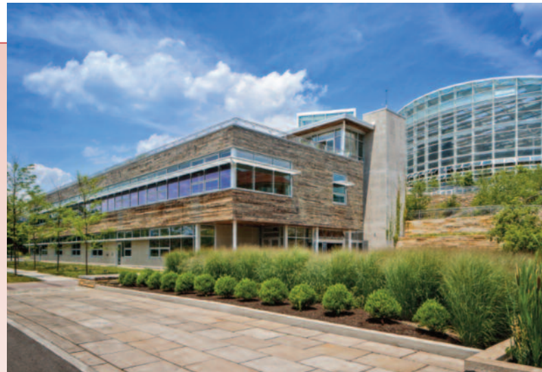
Phipps Center for Sustainable Landscapes. (Image: Denmark Photography Inc)
